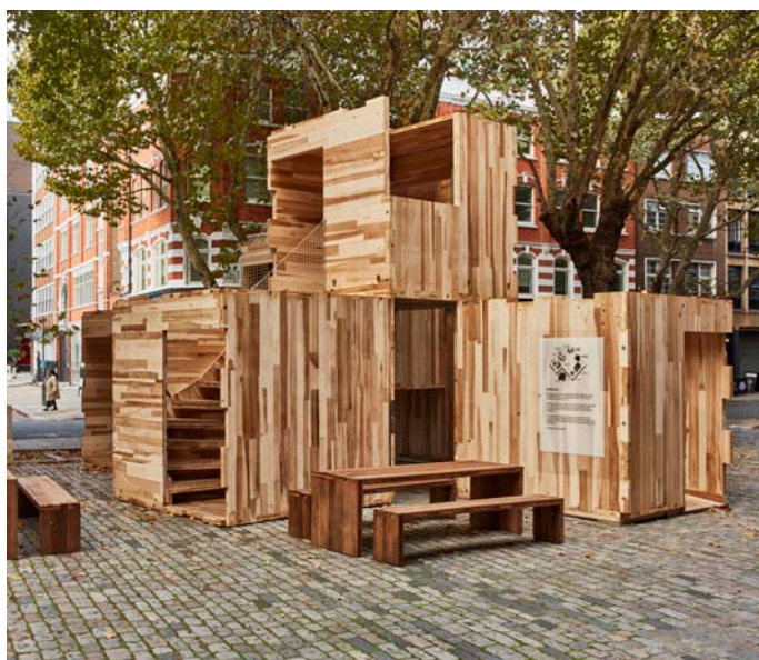
Six of the original seventeen tulipwood CLT modules outside the Building Centre.
